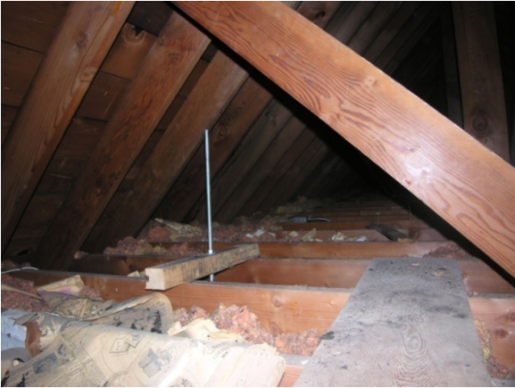
6. Roof framing over sanctuary
