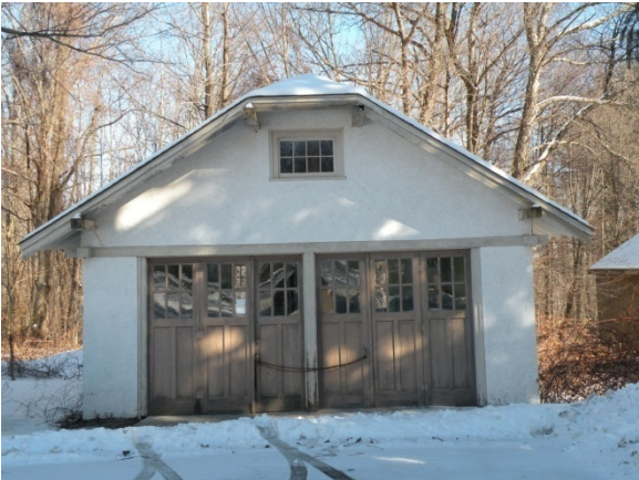
4. Separated garage front view
