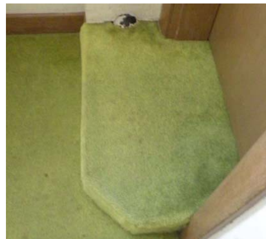
12. Step covering drain pipe in choir room
