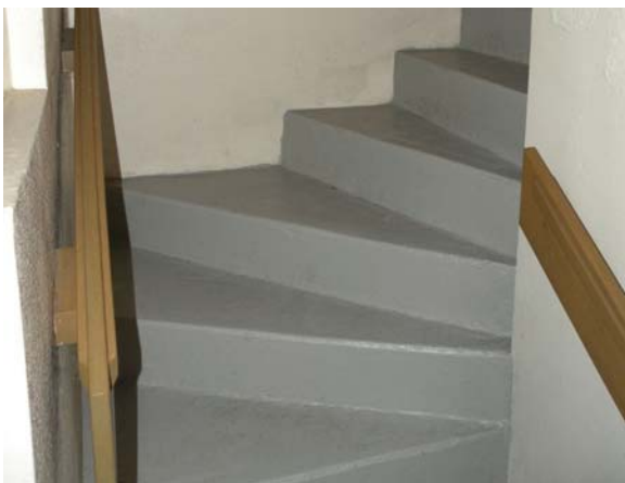
11. Stair winders to basement
