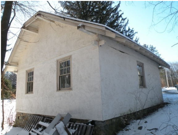
15. Rear view of separated garage
